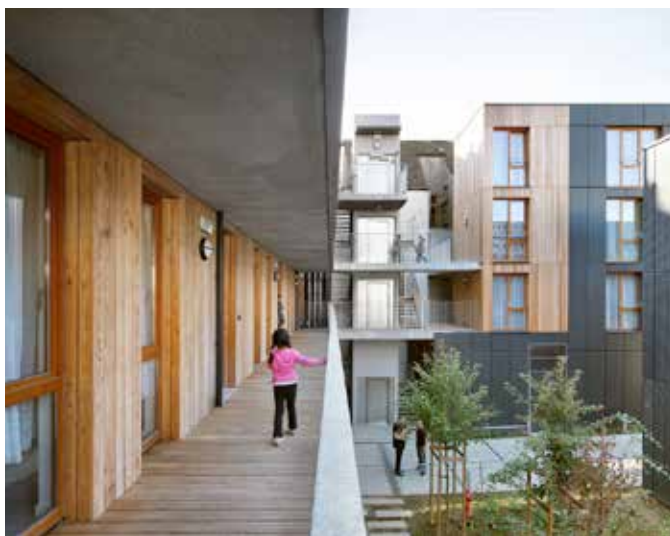
Savonnerie Heymans, Brussel, MDW Architecture
